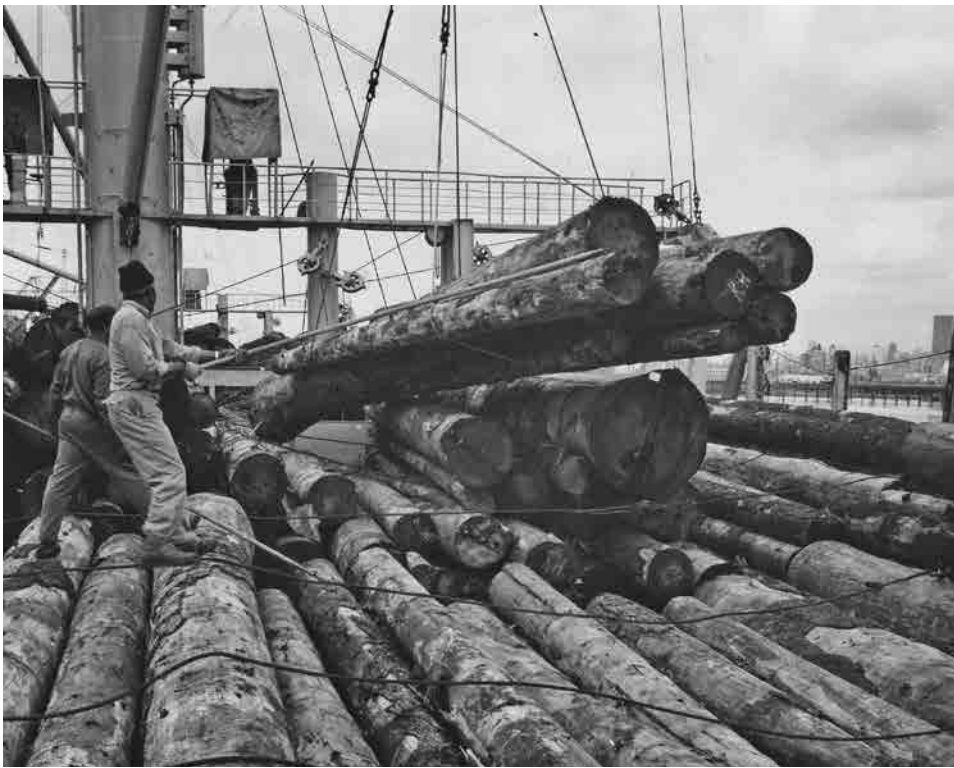
This photo taken in 1969 shows Local 19 members loading logs at the Port of Seattle's Terminal 105 using heavy lifts equipped with special gear. The technology of log loading changed quickly after 1959. Photo courtesy of ILWU Library and Archives.
